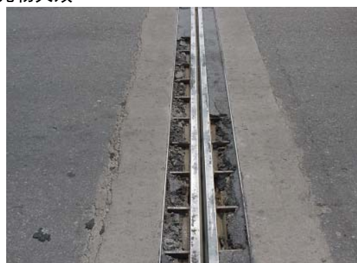
(b) 锚固区破损
