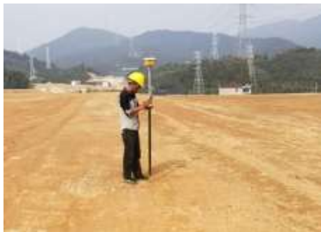
GPS放样中桩、边桩
