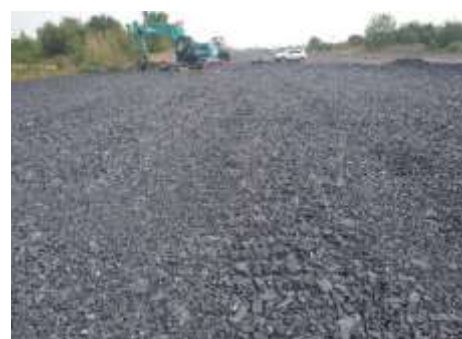
破碎后宕渣填筑
